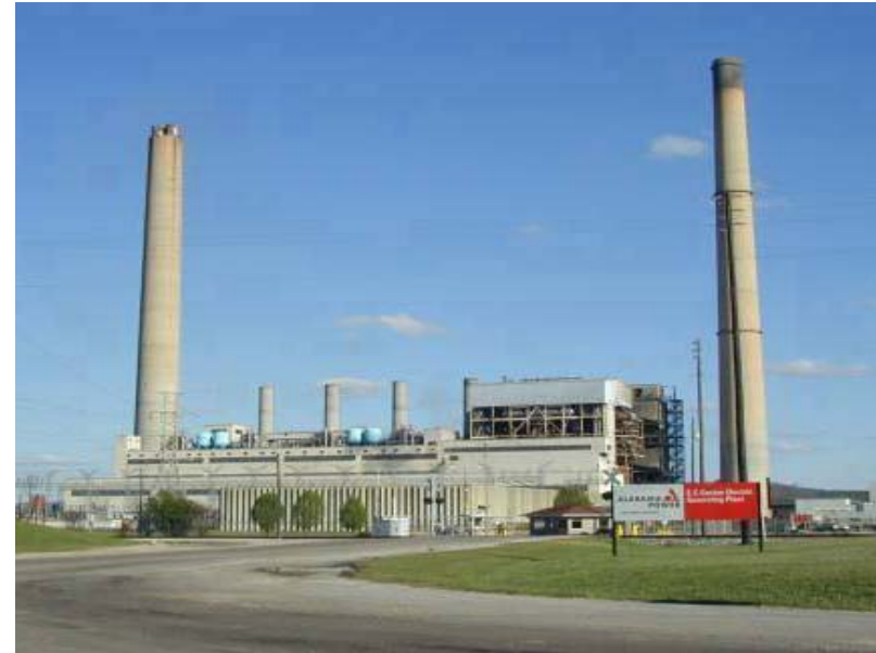
Alabama Power E.C. Gaston Plant
