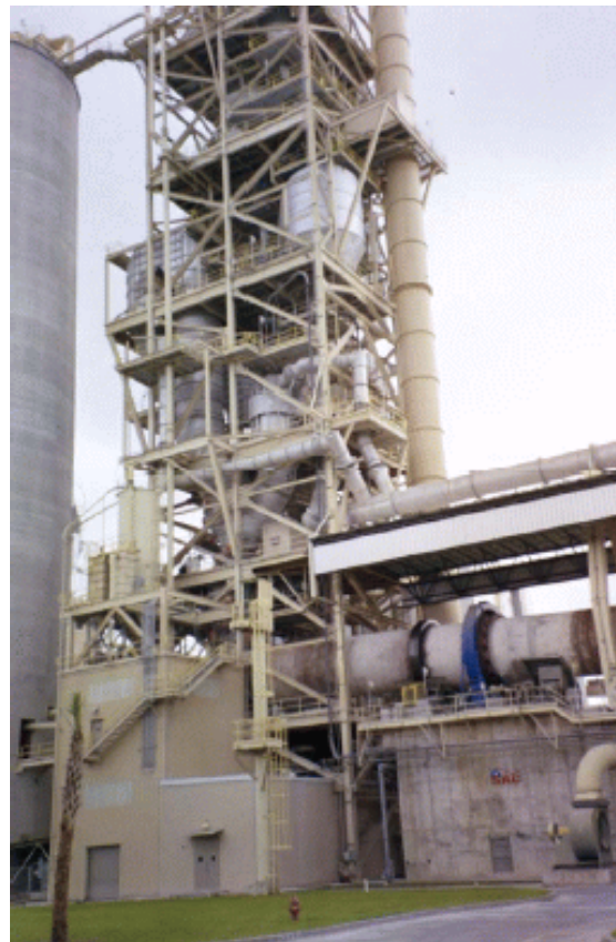
Figure 3-4. PH/PC kiln system.
