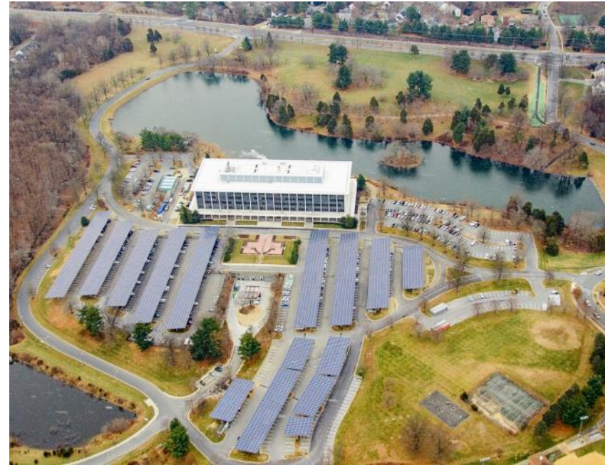
Montgomery County Public Safety Headquarter plans to install microgrids
