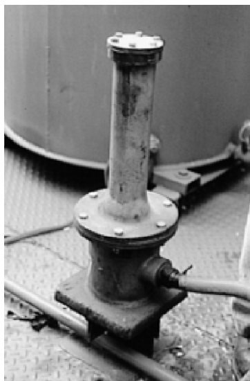
Figure 5-15. Roof-mounted rapper
