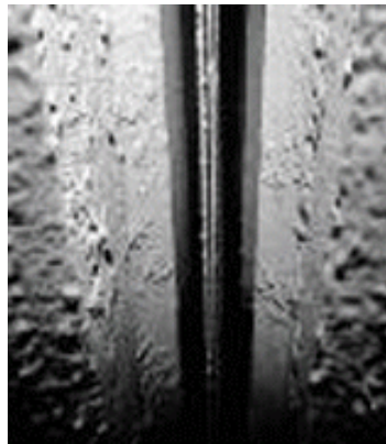
Figure 5-7. Gas passage between collection plates
