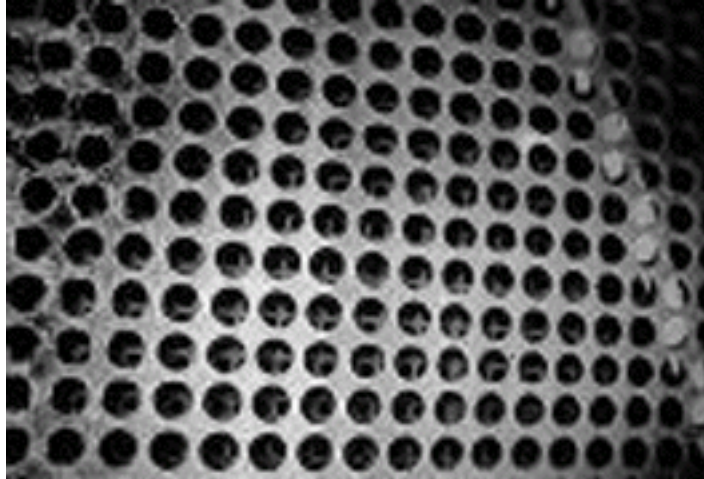
Figure 5-9. Gas distribution screens at the precipitator inlet
